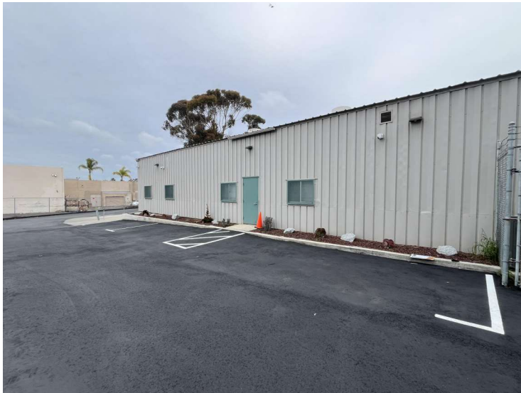
ENTRANCE TO LOWER OFFICE BUILDING - ENTRANCE DOOR'S LEVEL LANDING IS TOO STEEP AND DOES NOT PROVIDE COMPLIANT CLEAR FLOOR SPACE TAKEN 03/12/25
