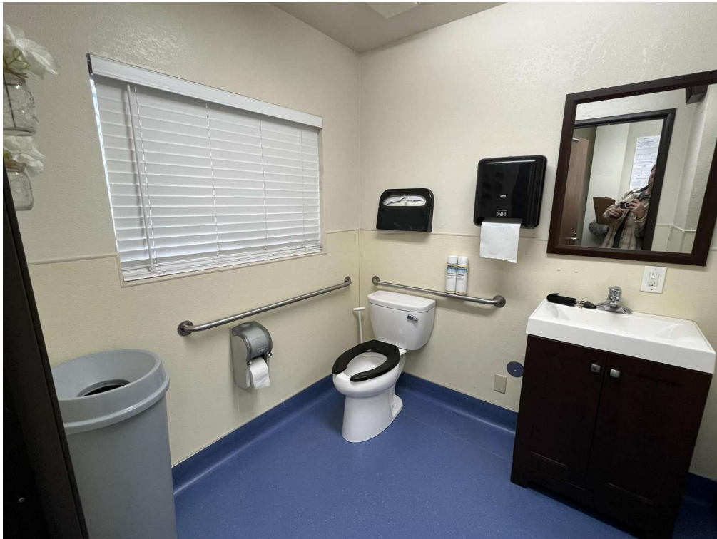
EXISTING RESTROOM - LAVATORY IMPEDES INTO THE WATER CLOSET CLEAR FLOOR SPACE AND WILL NEED TO MOVE TO SIDE WALL. RESTROOM ACCESSORIES WILL NEED TO BE REINSTALLED TO MEET CODE DIMENSIONS. WATER CLOSET LOCATION IS COMPLIANT. TAKEN 03/12/25
