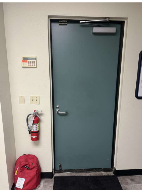
EXISTING OFFICE DOOR TO WAREHOUSE INTERIOR SIDE - DOOR SWING CAN BE REVERSED TO CORRECT CLEAR FLOOR SPACE ISSUE TAKEN 03/12/25
