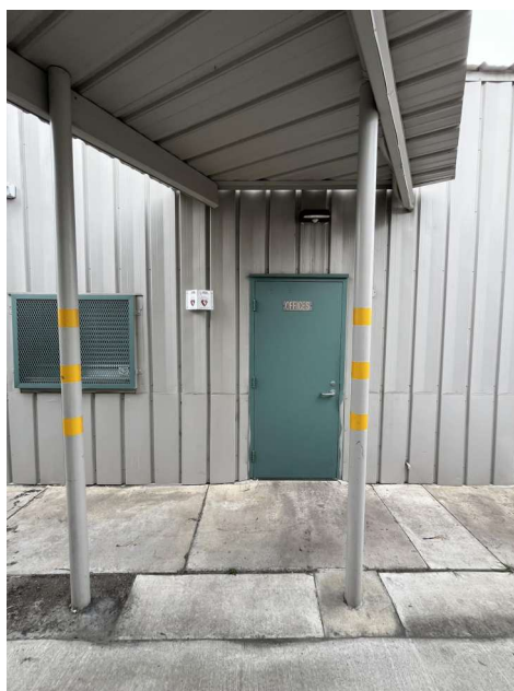
EXISTING OFFICE DOOR TO WAREHOUSE EXTERIOR SIDE - LEVEL LANDING IS TOO STEEP AND EXISTING COLUMN IMPEDES INTO CLEAR FLOOR SPACE TAKEN 03/12/25
